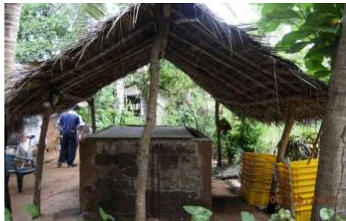
Fig. 1. Zero Energy Cooling Chamber (ZECC)
